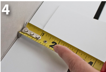
5 Place the side support strips. Place one support strip every 18". Offset about 1" forward so they are not touching the back wall
