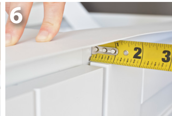
7 Cut the front edge strip to length, and align it with the inside edge of the front cabinet. It will extend beyond the cabinet to create 1.5" overhang
