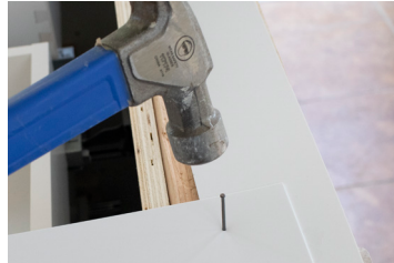
2 Tip: Use finish nails or glue to hold strips in place while you are templating
