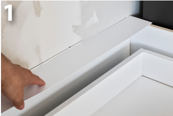
1 Cut back wall strip to length and lay it in place
